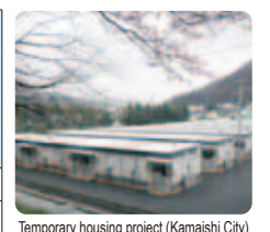
Temporary housing project (Kamaishi City)
