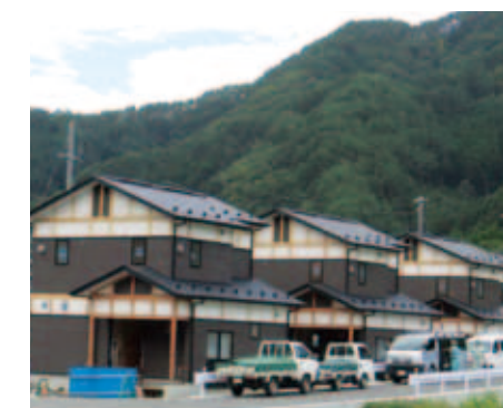
Public housing under construction (Otsuchi Town, September 2014)
